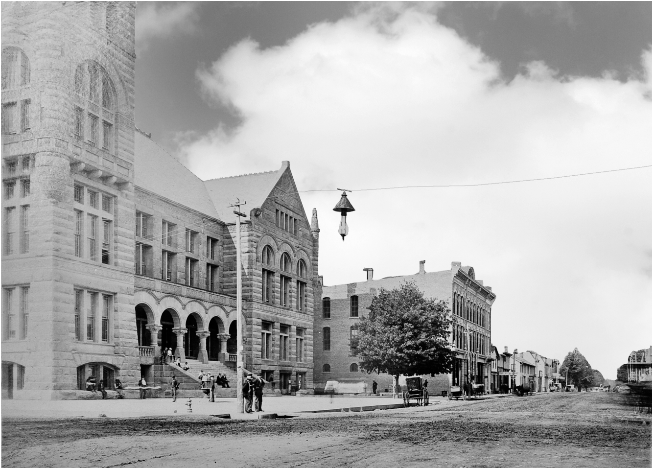
The 100 Block of West Market Street in Bluffton, Indiana in 1894.
