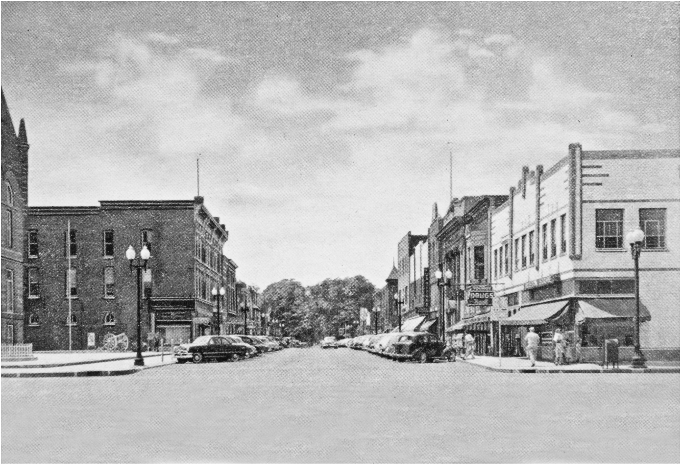
West Market Street in Bluffton, Indiana.
